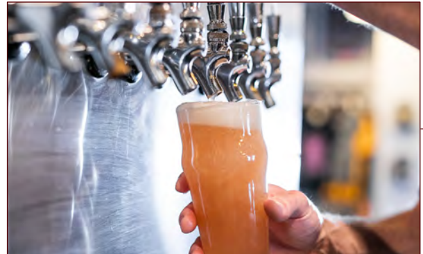
Figure 3.8. Properly balanced draught dispensing systems should deliver beer with a proper head.
