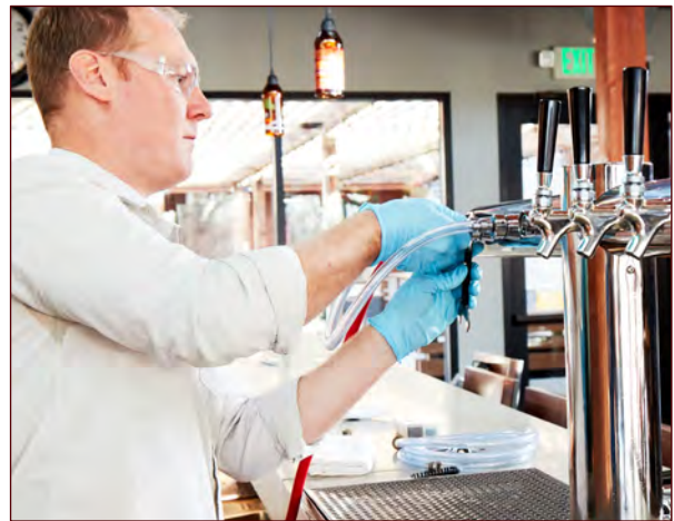
Figure 7.6. Proper PPE is necessary to prevent injury while cleaning lines.
